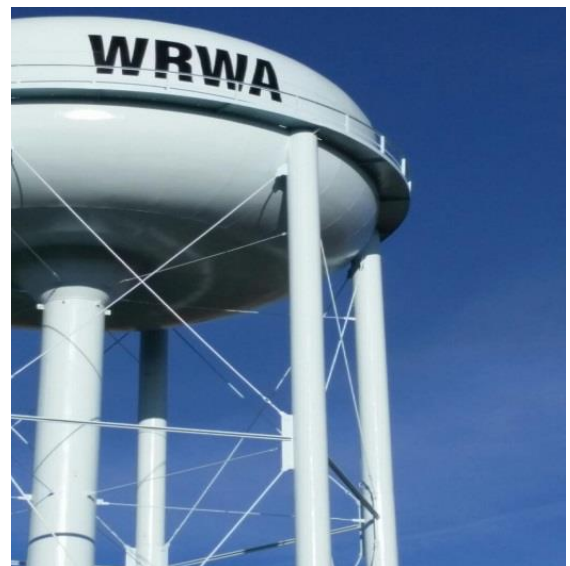
Fairfield Water Tower
